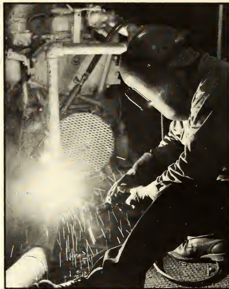
Figure 12.2. Heat and sparks from welding and burning operations could cause a fire if proper precautions are not taken.
