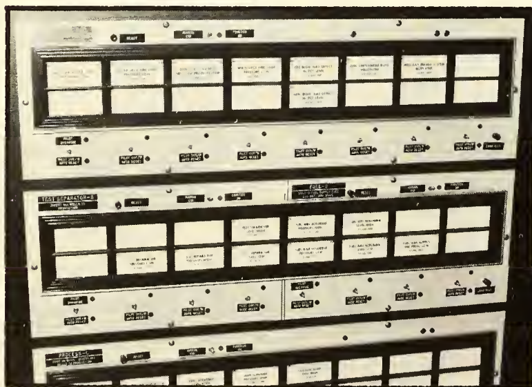
Figure 12.4. A central console is used to monitor all the fire loop systems installed on a rig.
