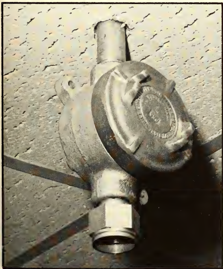
Figure 12.6. A combustible gas detector installed in living space. The detector senses the presence of flammable vapors in the surrounding air.
