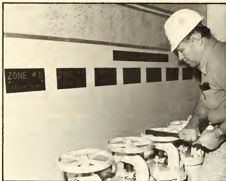
Figure 9.11. Zone valves and zone chart for a shipboard sprinkler system.
