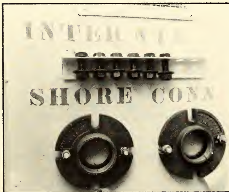
Figure 9.3. Portable international shore connection for ship's fire-main system.
